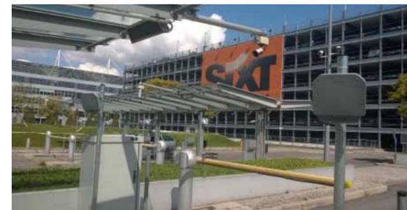
The latest generation of RFID Kathrein ARU4 series allows the rapid identification of vehicles
